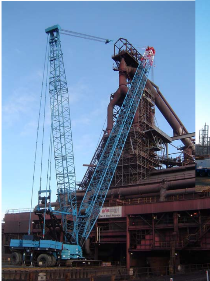
Above: M2250 Max-er working on a Blast Furnace in South Australia, Australia
